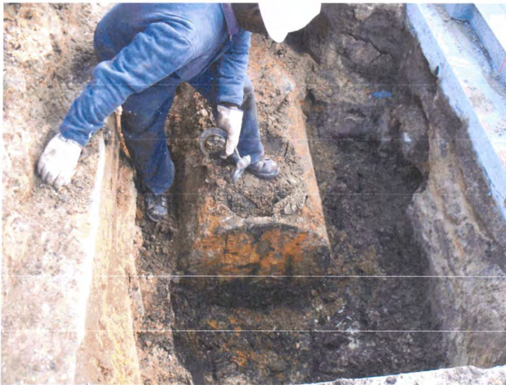
Picture 2: UST 1143Iris in the excavation before removal.
